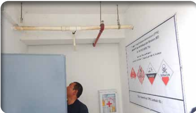
TPS Limbah B3 | B3 Waste Disposal Site
