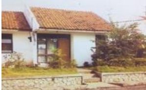
Jatiluhur Housing Authority employee residential complex, Purwakarta
